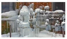
During Alaska's long winters, ice and snow can accumulate around the meter. Meters can be buried by snow falling from a roof or by snow plows. Additionally, be aware of icicles hanging from the roof, which can damage the meter when they fall.
